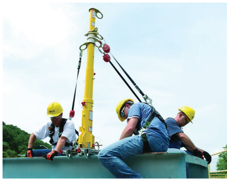
Telescoping design allows overall height to be adjusted in three stages from 0.83 m to 1.45 m (32.75 in to 57.25 in)
